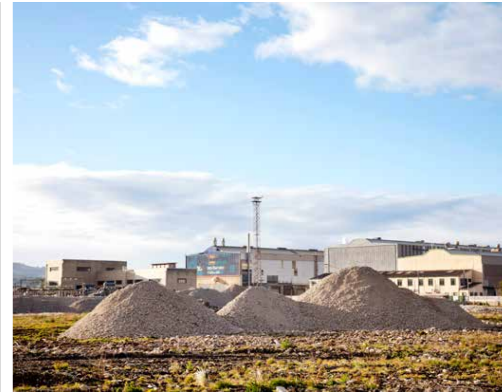
KiwiRail's old Hillside engineering workshops, which closed in 2012, with the remnants of the demolished Carisbrook Stadium in the foreground.
